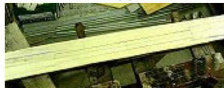
Again snap the edge centerlines. I’ve found that a quick stroke of the pull saw across the end at the level line makes a great notch to hook the chalkline into when repeatedly snapping these lines.
